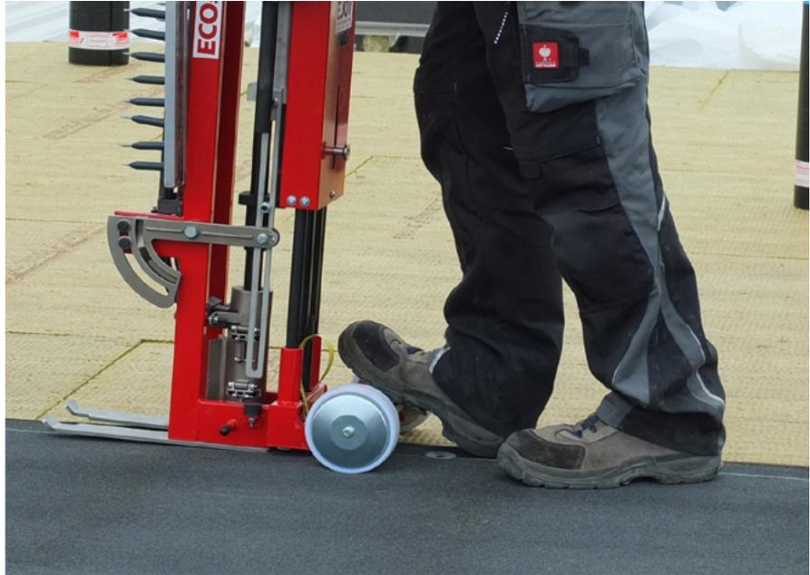
EJOT's ECOset HTK installation tool automates the fixing of the HTK 2G 50 tubewasher / fastener combination system. That means super-fast installation, better roof-top safety and greater all-round efficiency. EJOT is the first manufacturer to offer a battery powered installation tool, eliminating electric cables and tripping hazards. An additional cartridge holder is available, allowing up to 50 extra Dabo® fasteners to be housed.
