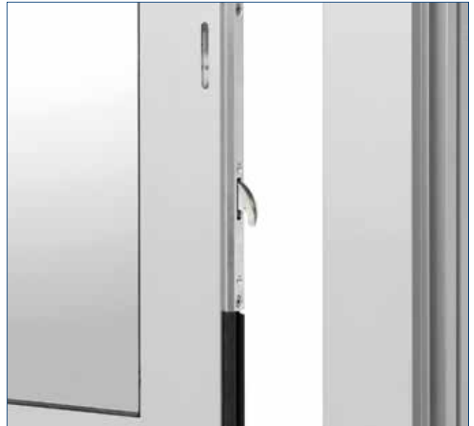
Lock A hook bolt lock installed
