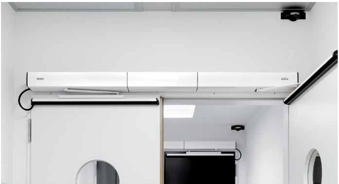
TSA 160 NT Z-IS, radar movement detector and GC 302 / GC 334 sensor strips, Andels Hotel, Berlin, Germany (photo: Stefan Dauth / GEZE GmbH)
