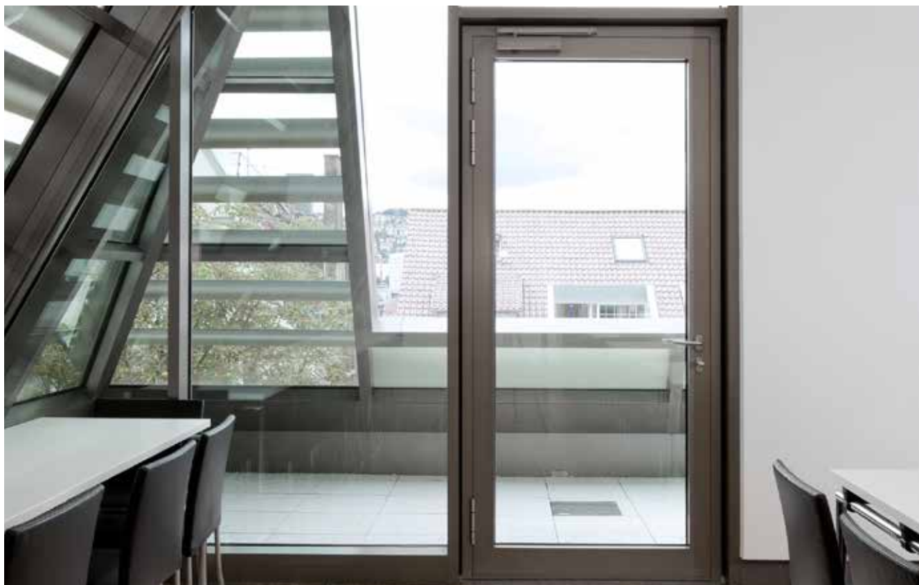
TS 5000 with T-Stop guide rail, Catholic Church Administration Building, Stuttgart, Germany (photo: Dirk Wilhelmy)
