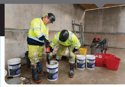
When mixed with clean water and applied correctly, **Tanking Slurry** forms a permanent waterproof coating to the concrete and masonry and is easily applied by brush, roller or spray.
