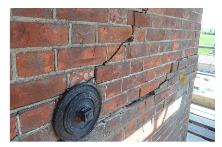
This technique generates an in situ reinforced, deep masonry beam. In order for the reinforced beam zone to accommodate the imposed flexural forces, it is necessary to repoint loose mortar joints and to deep-resin-inject cracks with an appropriate resin or grout.
