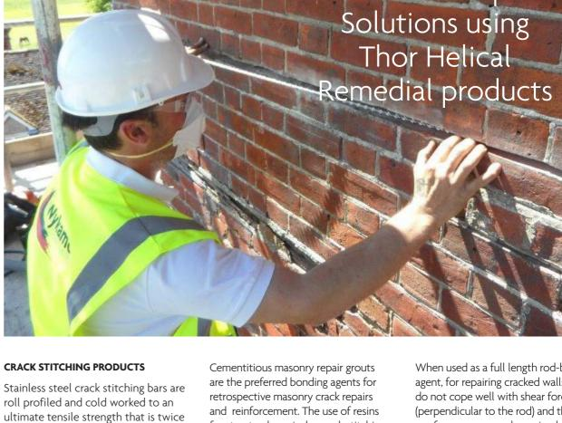
roll profiled and cold worked to an that of rebar, four times that of epoxy glass-fibre rods and seven times that of flat twisted plate [ref: BRE GBG 62].
