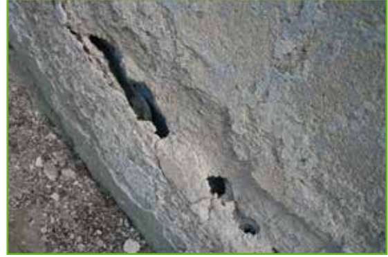
Damaged plaster / render
