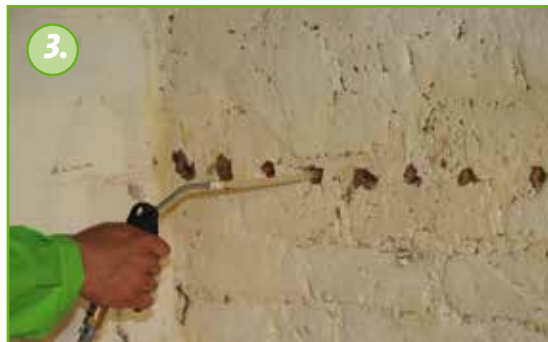
The boreholes are cleaned from dust by blowing the dust out of the borehole with pressurised air.
