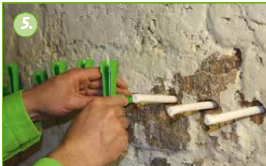
The KÖSTER Suction Angles are installed so that the KÖSTER Capillary Rods reach into the supply chamber of the KÖSTER Suction Angles.
