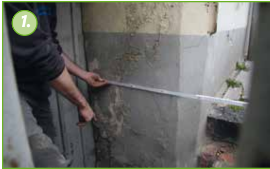
The masonry is from 1750, the existing plaster is damaged. The salt and moisture contents are high.
