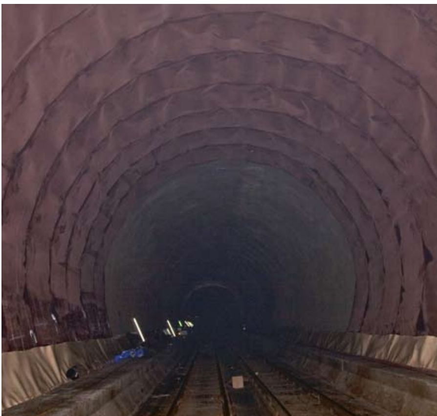
View of the Gotthard tunnel with DELTA®-AT 1200 installed.
