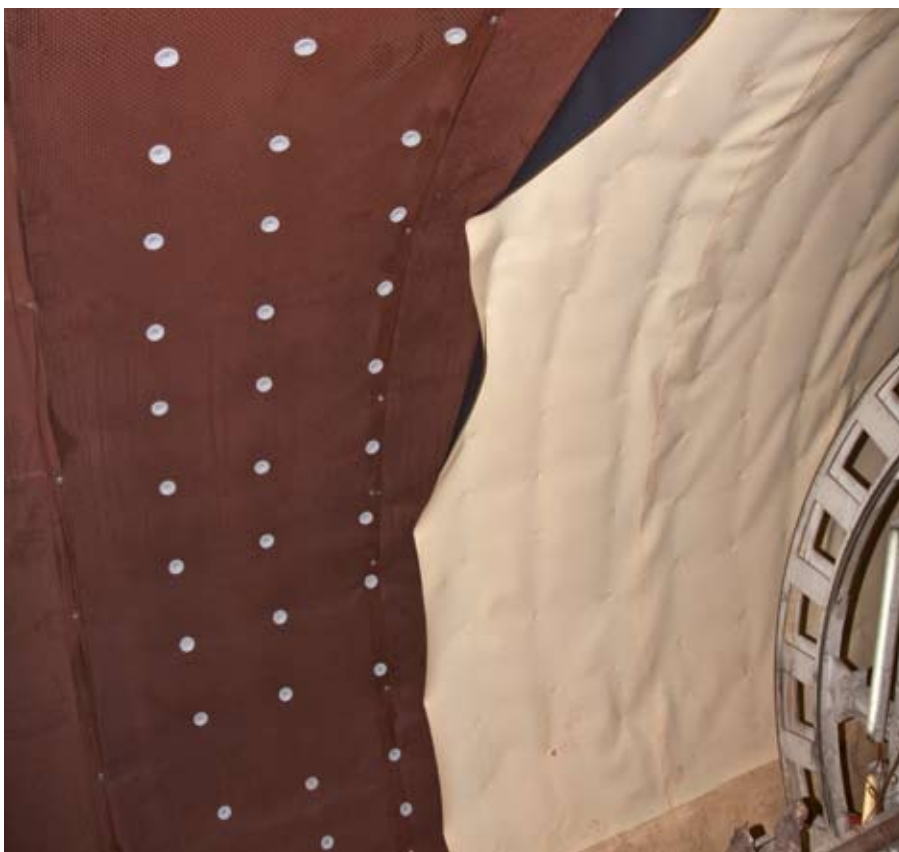
Additional fastening by washers to which the waterproofing will be welded later on.
