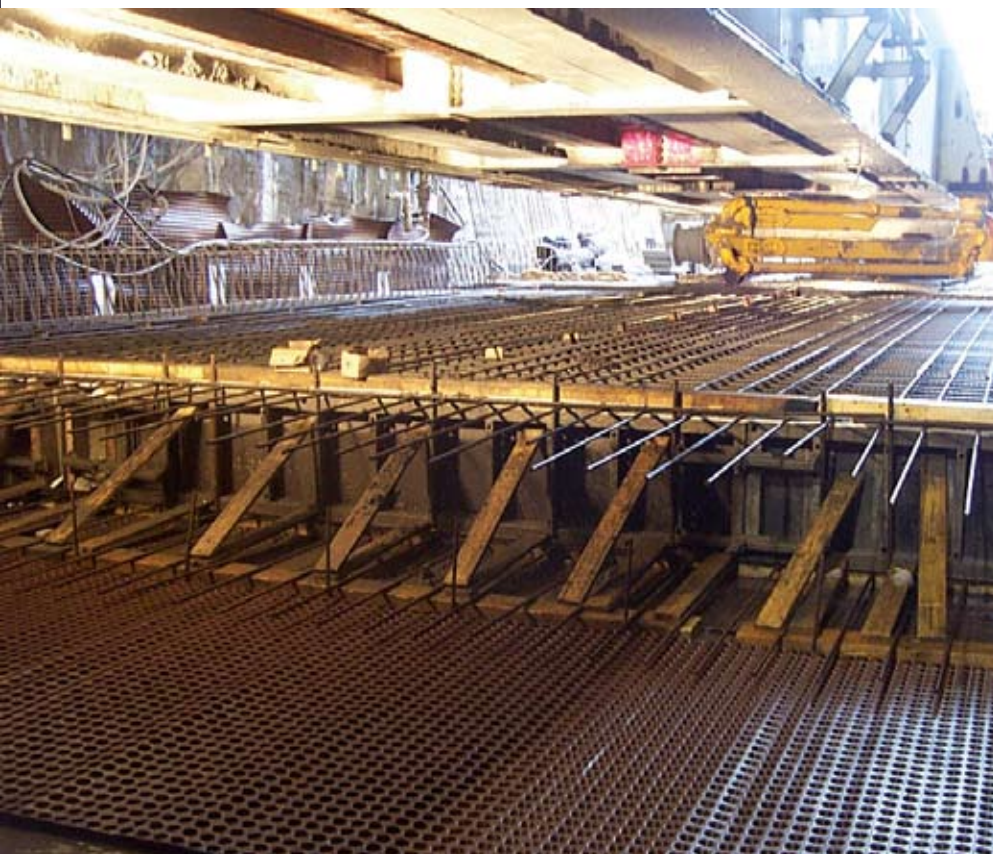
DELTA®-MS 20 to protect the tunnel floor.
