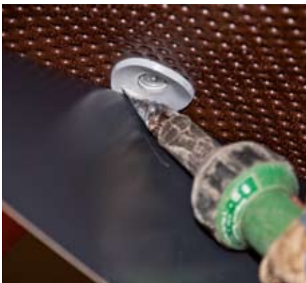
Welding the waterproofing layers to the washers.
