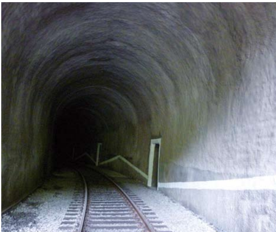
The new inner shell of reinforced shotcrete.
