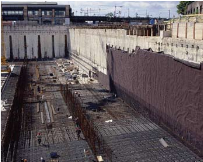
■ 16 Example: diaphragm wall application in Duisburg.
