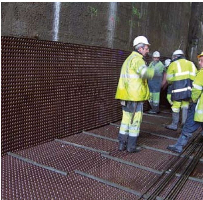
Sheets laid out double along joints.
