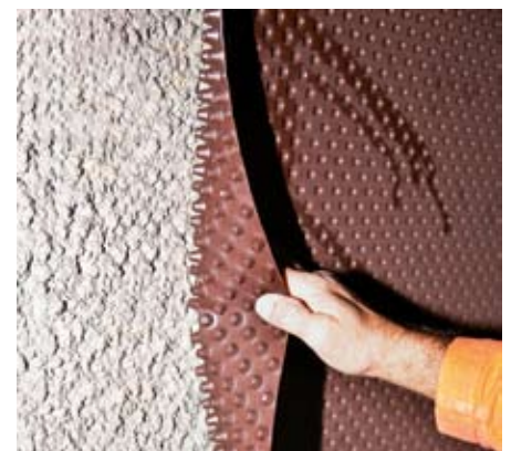
Drainage sheet atop a shotcrete inner shell.
