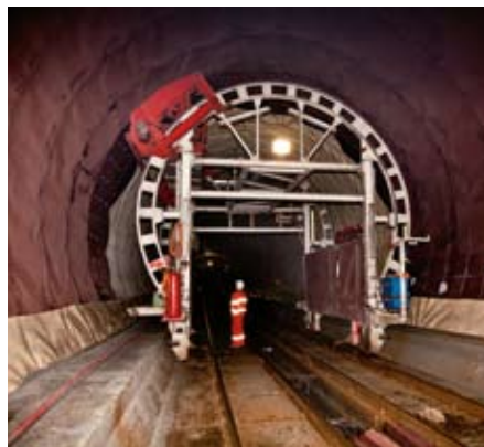
Sheets being fastened directly from the installation truck.
