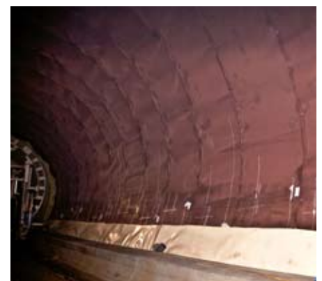
Initially, sheets are fastened only in the overlap zones.
