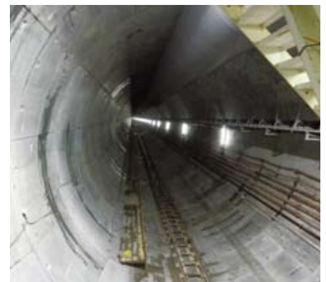
Leaks before the application of a drainage sheet.
