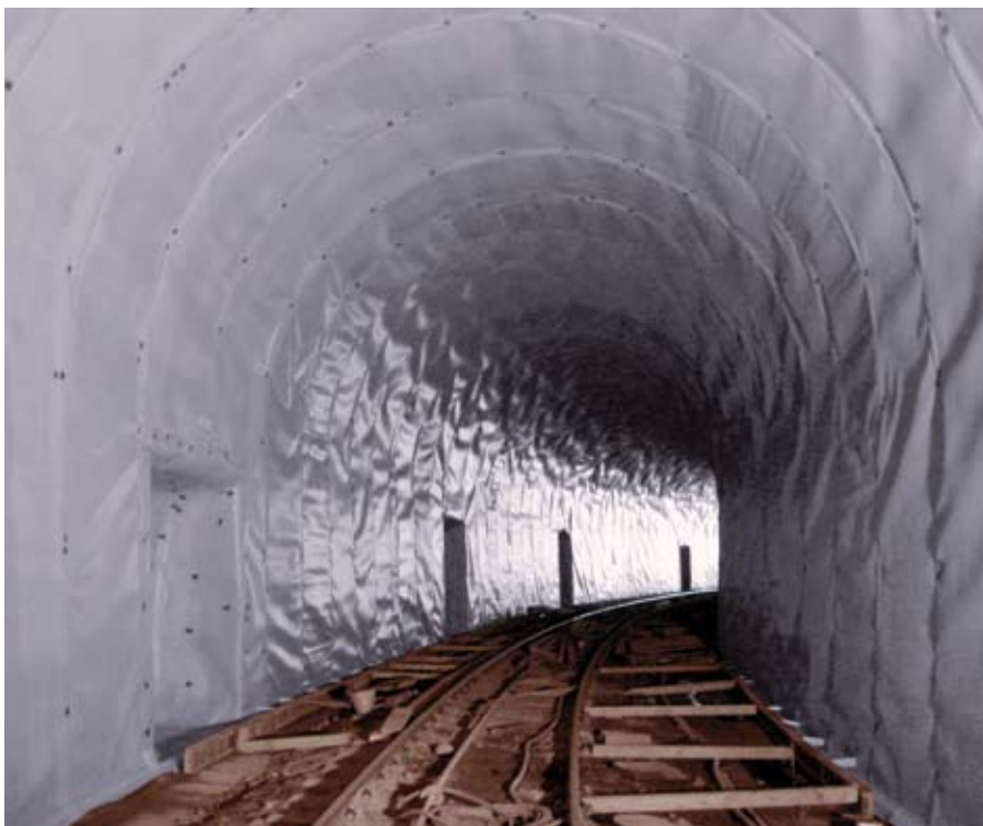
The railway tunnel complete with DELTA®-PT lining.
