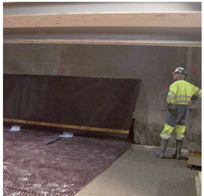
DELTA®-MS 20 on the floor, DELTA®-MS on the wall.
