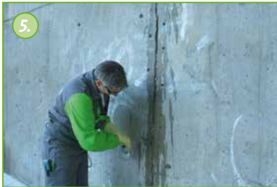
Pre-wet the crack.
