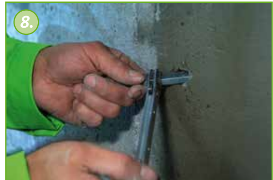
Use a wrench to tighten the packer.
