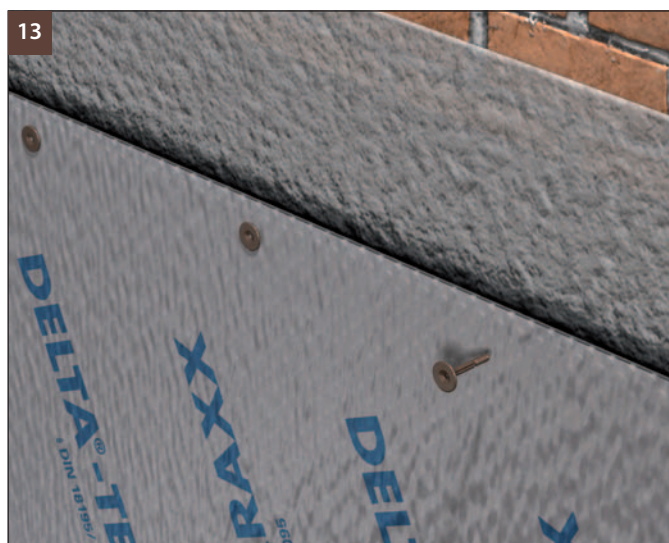
(Fig. 13) If the grade line is known, the sheet may be fastened immediately using DELTA ® -MS DÜBEL.
