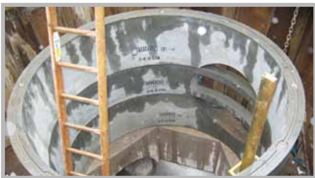
3000mm sectional chamber installation with a letter box opening for 1500mm concrete pipe
