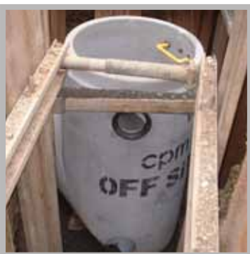
1200mm stop end bend complete with high level inlet
