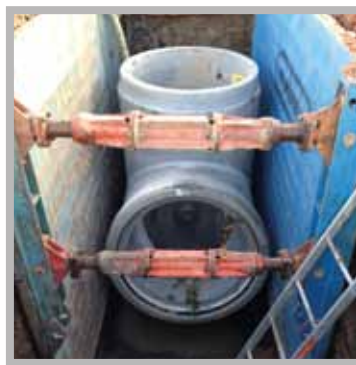
1200mm end entry manhole complete with hydrobrake
