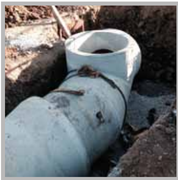
900mm off 900mm mid entry manhole
