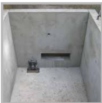
Once-piece chamber with inlet and outlet holes
