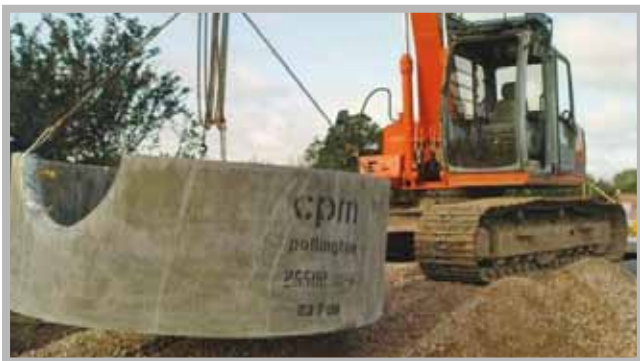
2550mm sectional installation, base chamber complete with half formed hole for 750mm pipe
