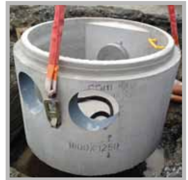
1800mm sealed chamber complete with Optimum Hydro-Brake®
