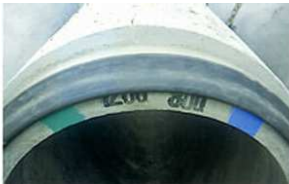
View of correctly positioned seal
