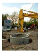
Marshalls CPM offer reinforced precast concrete manhole units specially designed for sinking by using by the caisson method. This is achieved by using a shaft sinking plate system and is widely used for construction of pumping station, wet wells and manholes, particularly in difficult ground conditions.
