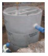
The Downstream Defender<sup>®</sup> is an advanced hydrodynamic vortex separator for the effective and reliable removal of fine particles along with oils and other floatable debris from surface water runoff.
