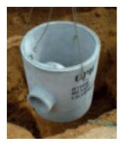
The Hydro-Brake Optimum<sup>®</sup> chamber comprises of a precast concrete chamber base containing a bespoke Hydro-Brake Optimum<sup>®</sup> Flow Control which is delivered to site ready for immediate installation.
