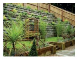
Each block weighs approximately one tonne and is dry laid. Walls can be built in a fraction of the time and cost compared with other methods. Due to the dome and groove joint – straight or curved walls can be constructed. Redi-Rock<sup>™</sup> concrete blocks from Marshalls CPM offer quality sustainable solutions for many applications.
