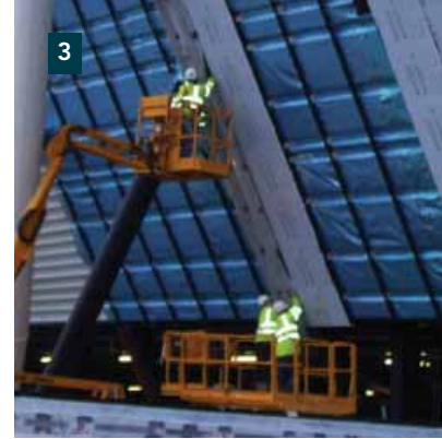
3. Olympic Stadium – manufacturing machinery was transformed to cope with the World's longest sheets of Alpolic material and a full size rig constructed to test handling, transport and application.
