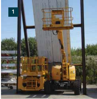
1. A full-size test rig was built to ensure the record breaking panels could be transported, handled onsite and fixed without problems.
