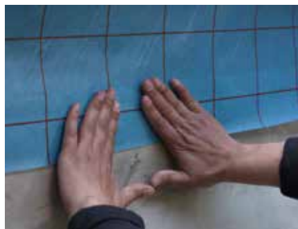
8. Fold DuPont™ AirGuard® AVCL onto primed surface
