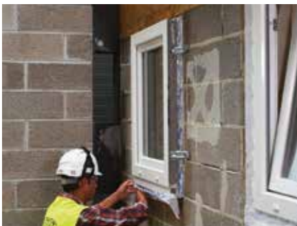
4. Fit the tape to the window cill first and press firmly into place
