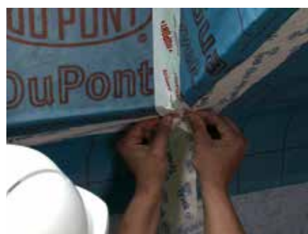
18. . . . a flexible tape that can be used to seal corners and any awkward details
