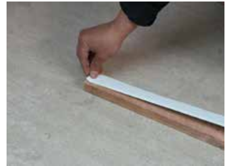
12. Apply Tyvek® Butyl tape to batten
