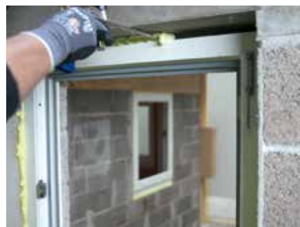
3. Repeat the process from inside the building
