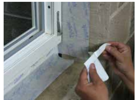
9. Remove the release paper from the back of the tape
