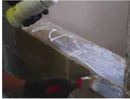
2. Apply primer also to the window head, cill and reveals
