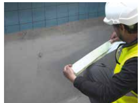
9. Prepare Tyvek® Plastering Tape by folding back along the first split liner
