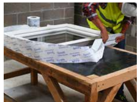
6. Repeat the same procedure as for the exterior side of the window. This time remove the large release liner of the tape (6 cm) and apply Tyvek® Plastering Tape to the window frame
