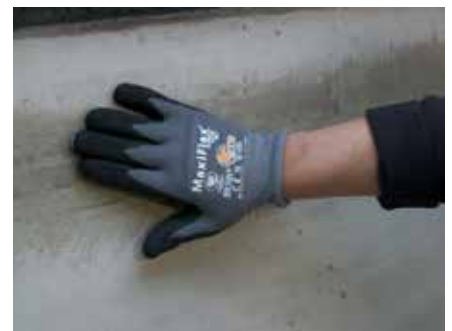
6. After an hour the primer turns transparent
