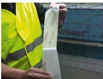
17. Remove release liner from DuPont™ AirGuard® Tape . . .
