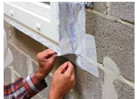
9. ...and dress around window frame, pressing firmly into place
