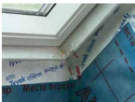
16. Cut tape may be used to seal internal corners
