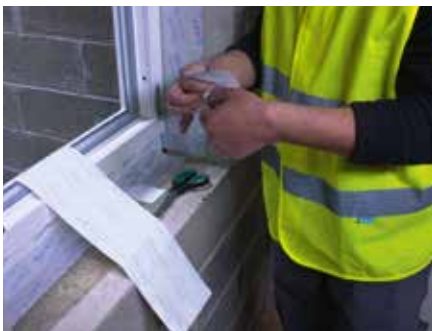
7. Fold and stick the tape to form a small corner detail...
