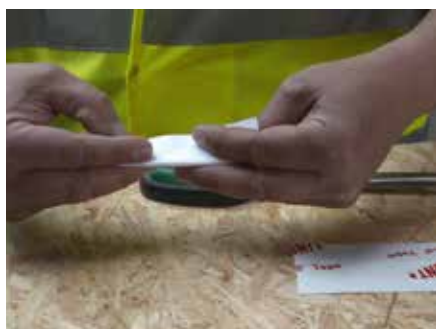
13. Fold DuPont™ AirGuard® Tape in half
