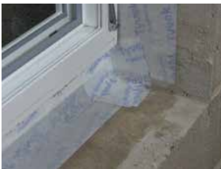
10. Position and firmly press the corner detail into place
