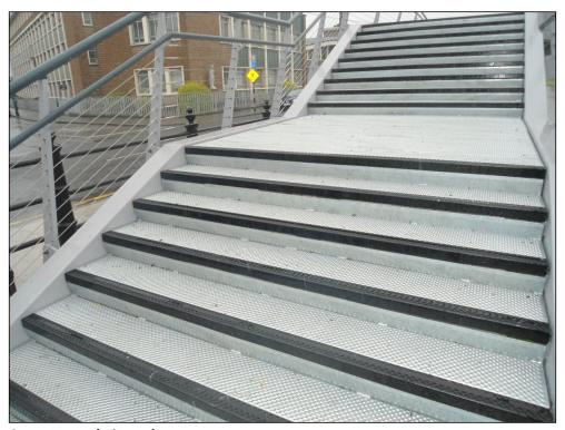
**Stair Treads/Landings** Type O5-M - Treads 2500x325mm including Cranked Rear Riser (Galvanised with Polyester Powder Coated Nosing)
