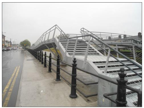
**Stair Treads/Landings** Type O5-M - Treads 2500x325mm including Cranked Rear Riser (Galvanised with Polyester Powder Coated Nosing)
