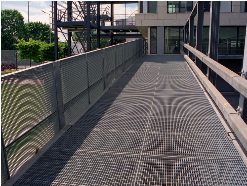
Walkways, Balustrade Infills
