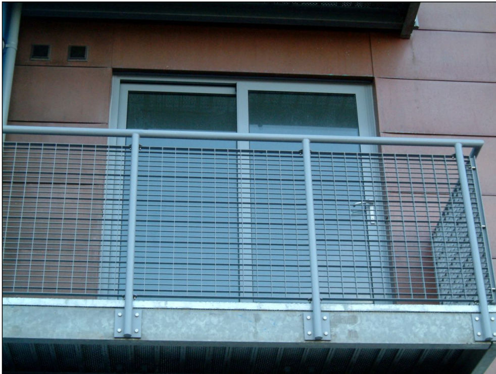
Balustrade Infills, Balconies
