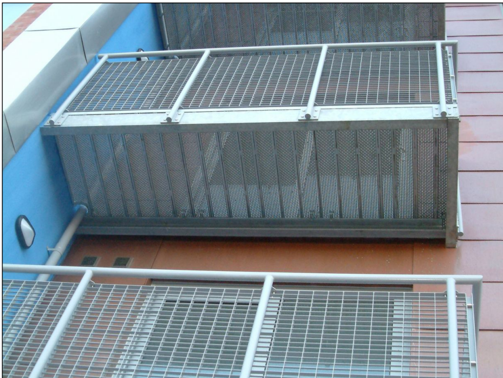
Balustrade Infills, Balconies
