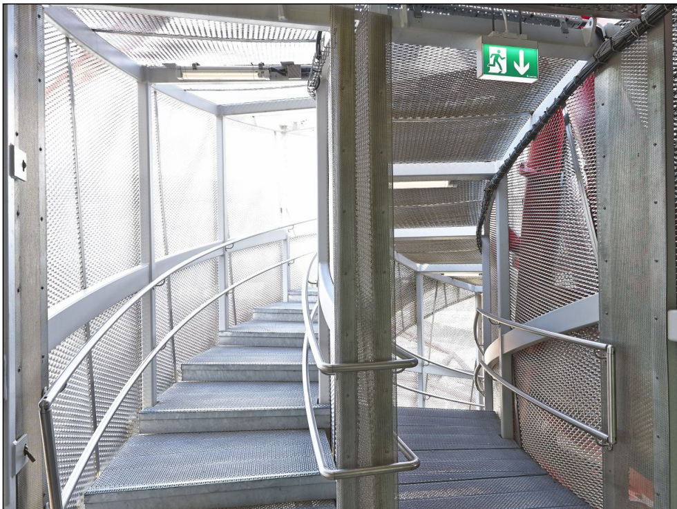
Walkways, Stair Treads/Landings
