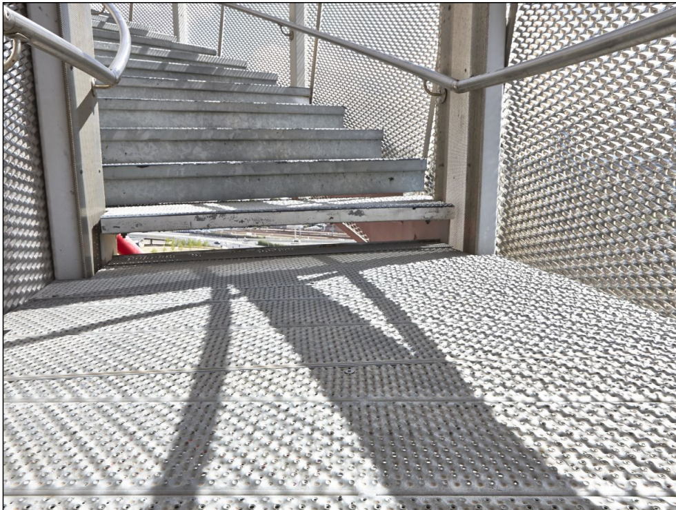
Walkways, Stair Treads/Landings
