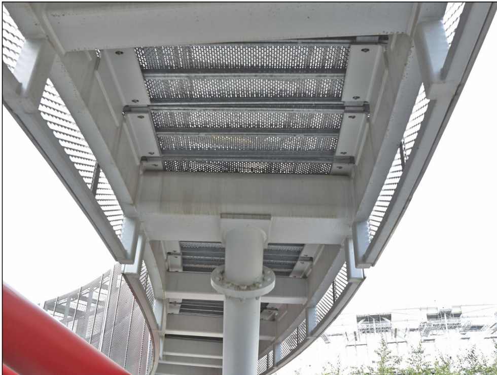
Walkways, Stair Treads/Landings
