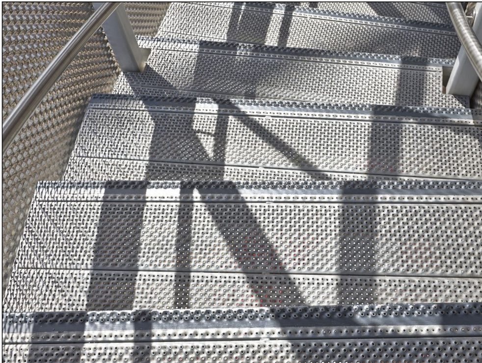
Walkways, Stair Treads/Landings
