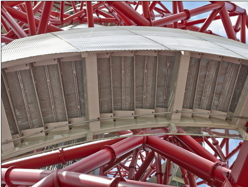
Walkways, Stair Treads/Landings
