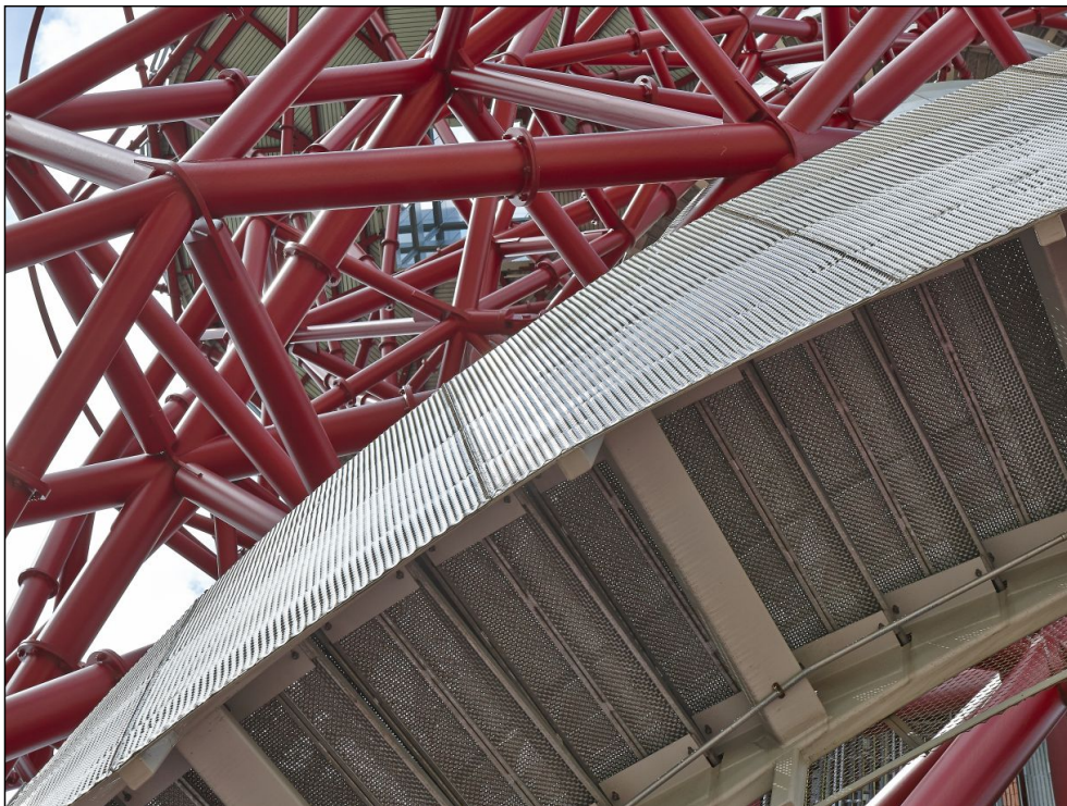
Walkways, Stair Treads/Landings
