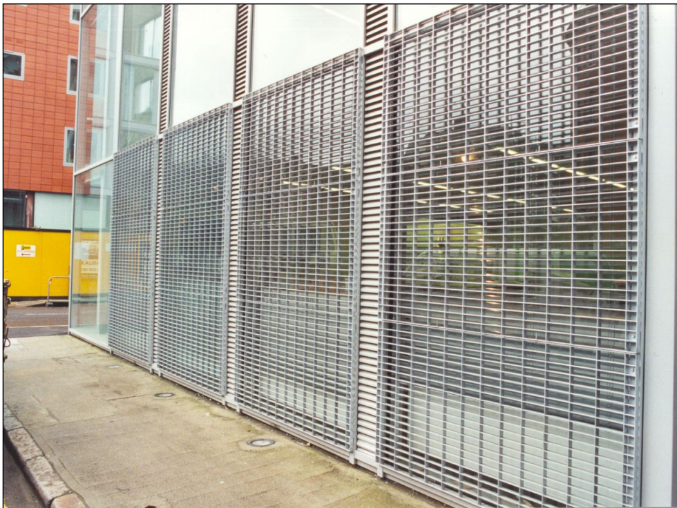
Screening/Fencing, Brise Soleil Type N - 150x50/30x3N/30x3mm (Galvanised)
