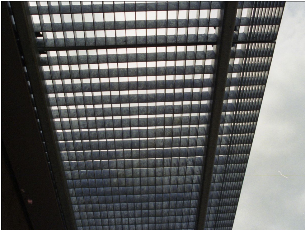
Walkways, Brise Soleil
