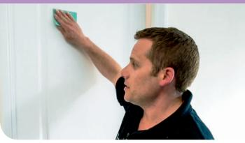
2. Brush off prepared surface to remove dust
