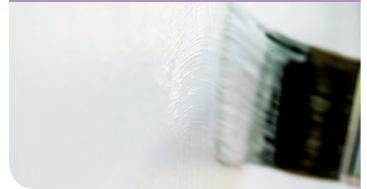
**3.** Lay the paint off to remove any brush or roller marks
