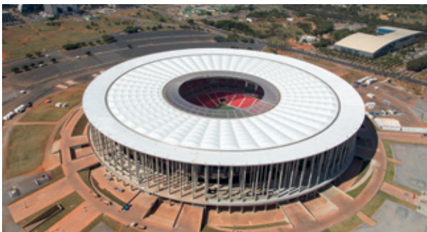
Estádio Nacional, Brasília: TROX ventilation and air conditioning in all newly built World Cup stadia in Brazil
