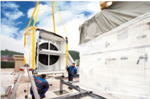
Delivery and installation of a weatherproof X-CUBE
