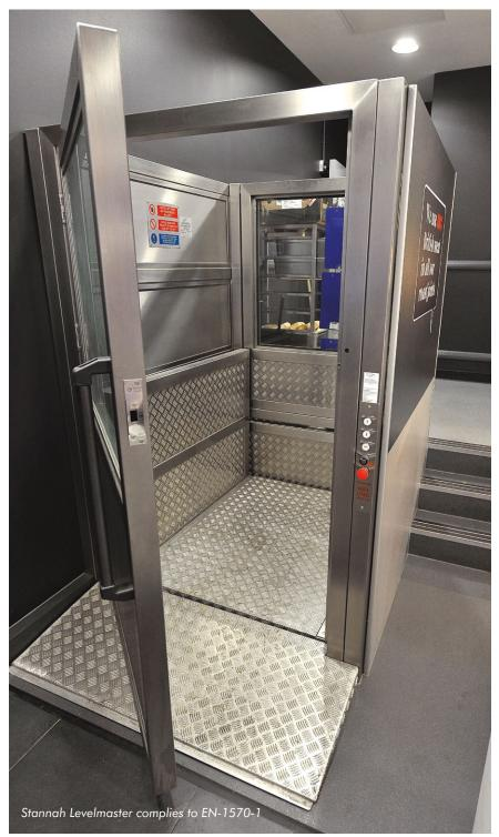
Levelmaster is an ideal solution where goods need to be moved over a small change in level. It offers a cost-effective, simple solution with a wide range of platform sizes.
