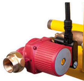
Secondary Pump HWS Transfer (+1T)
