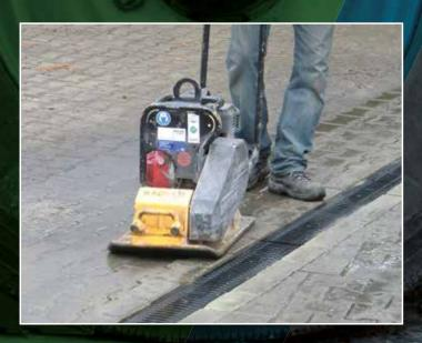
Elasticity is important when permeable paving surfaces are being compacted in along the **RECYFIX** channel.
