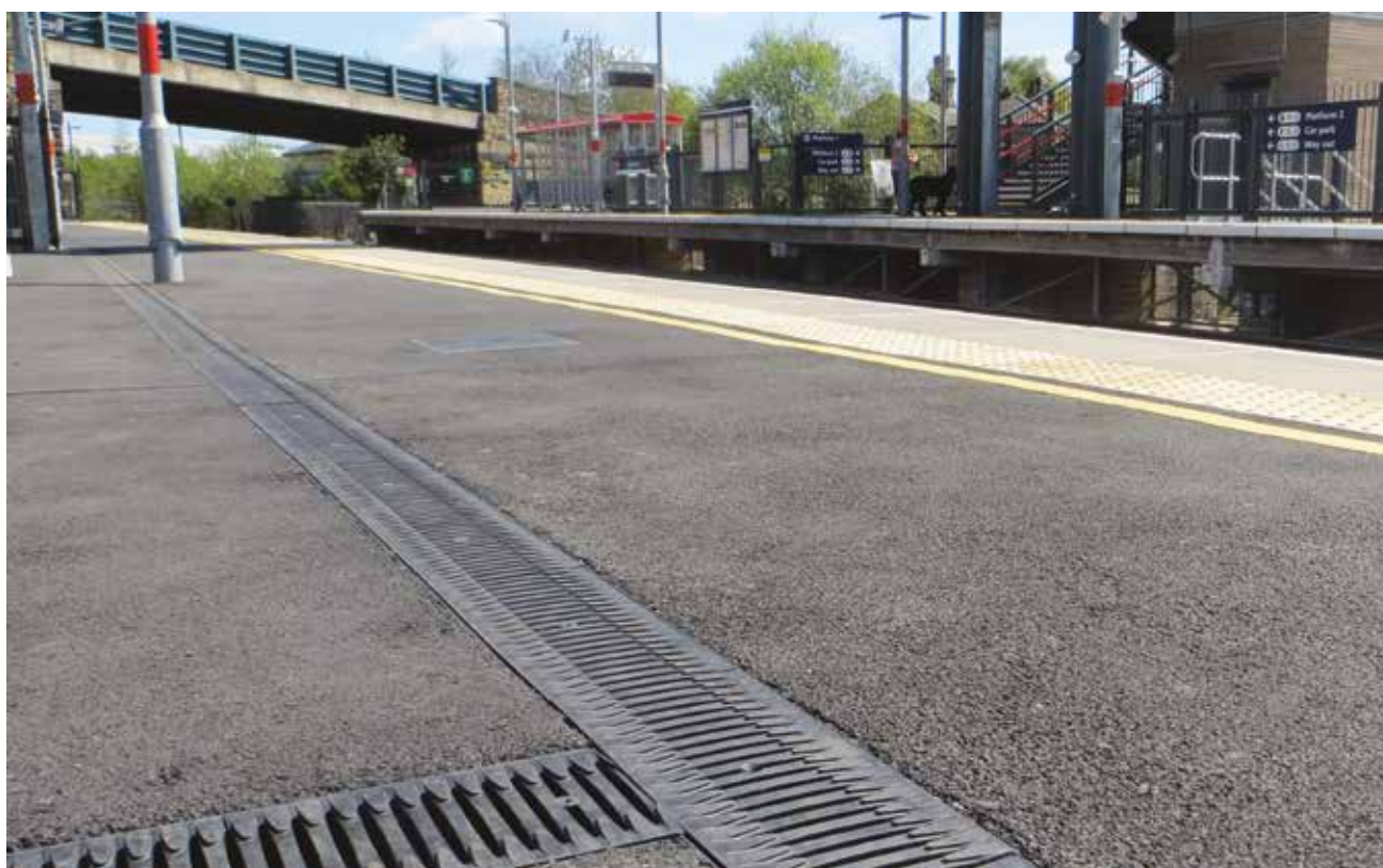
Low Moor Railway Station, Bradford
