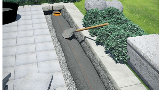
Fill with concrete and compress to foundation.
