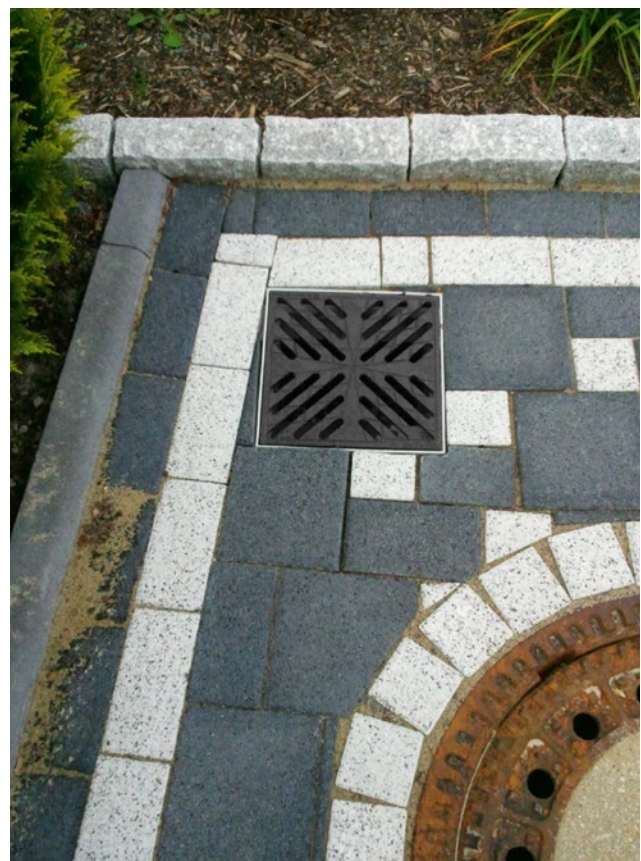
Private house in Wiehl, Germany
