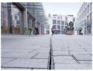
Surface drainage with tailor-made slotted channels.
