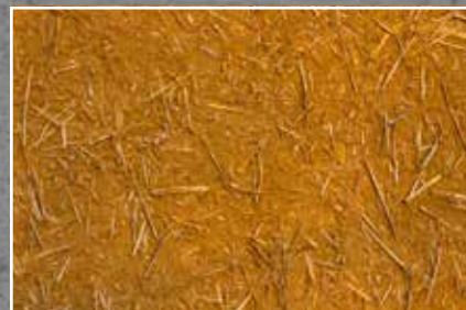
Clay wall reinforced with plant fibres.
