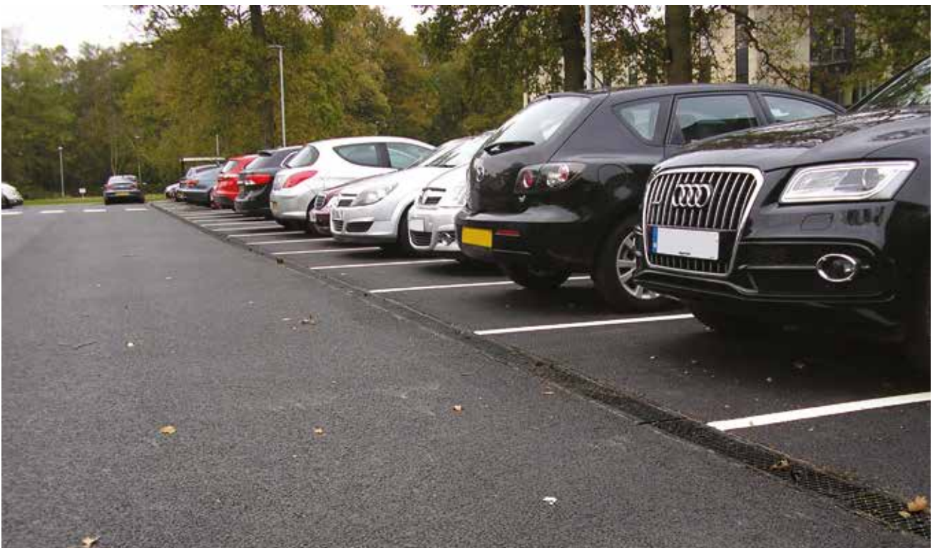
Fire Brigade Training Centre Car Park Moreton
