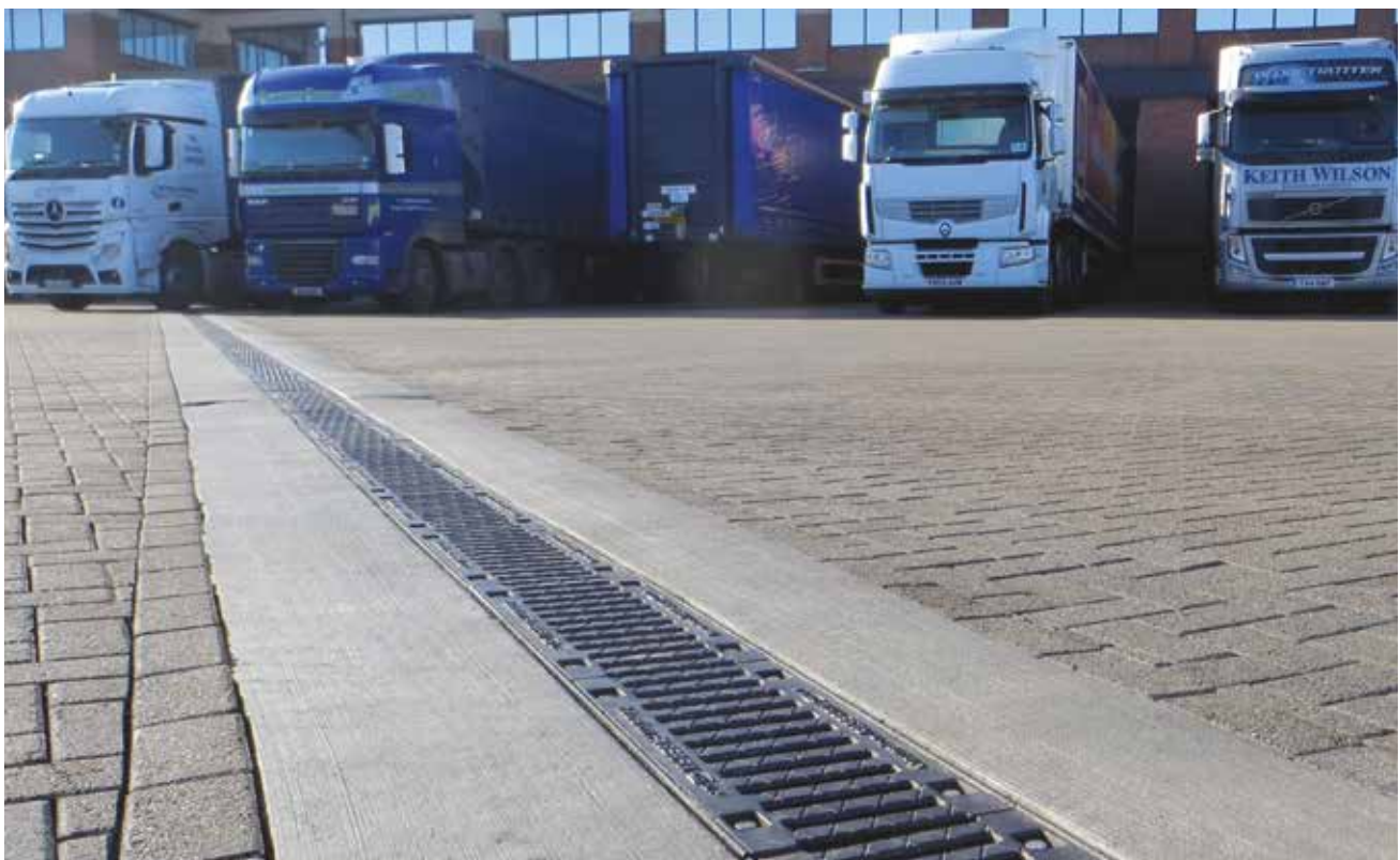
ALDI Regional Distribution Depot Darlington
