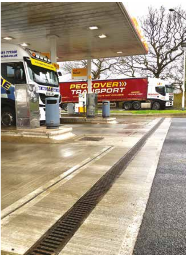
Charnock Richard Services HGV Refuelling Station
