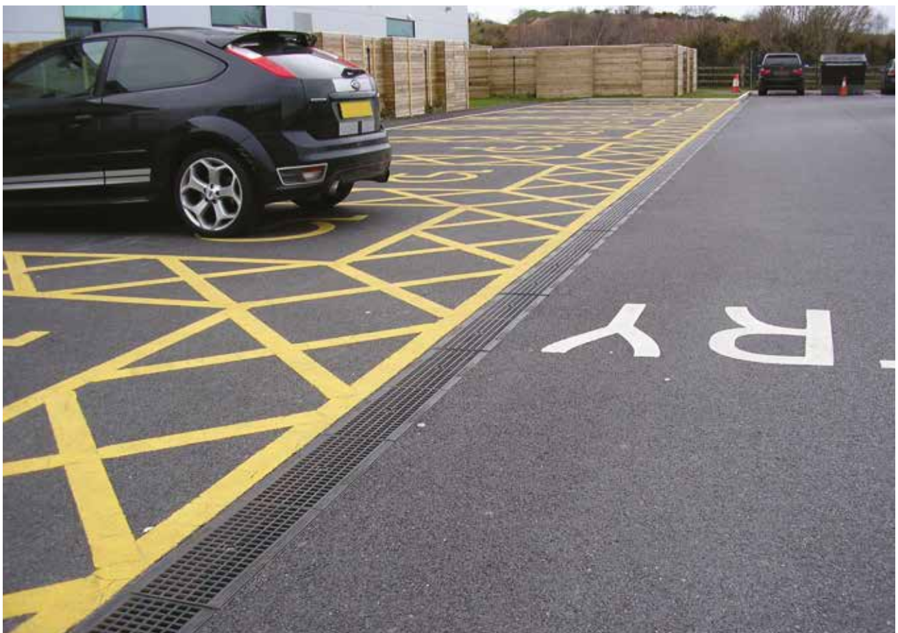
Car Park Exeter
