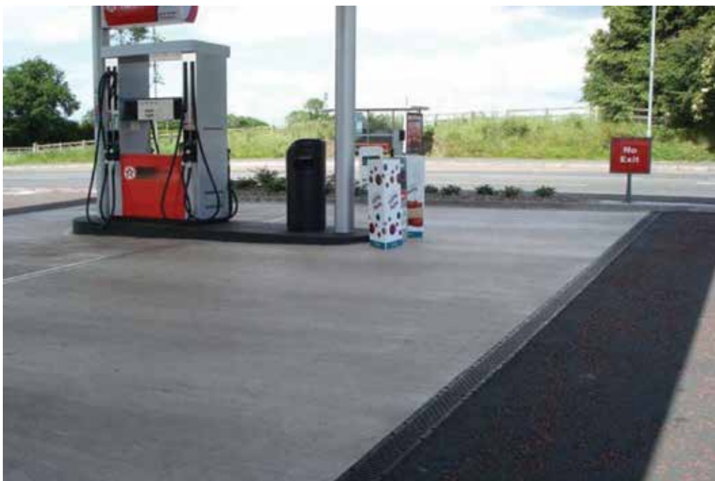
Petrol Filling Station
