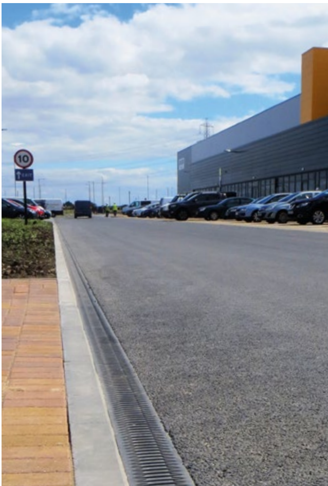
AMAZON regional distribution centre, Doncaster, United Kingdom
