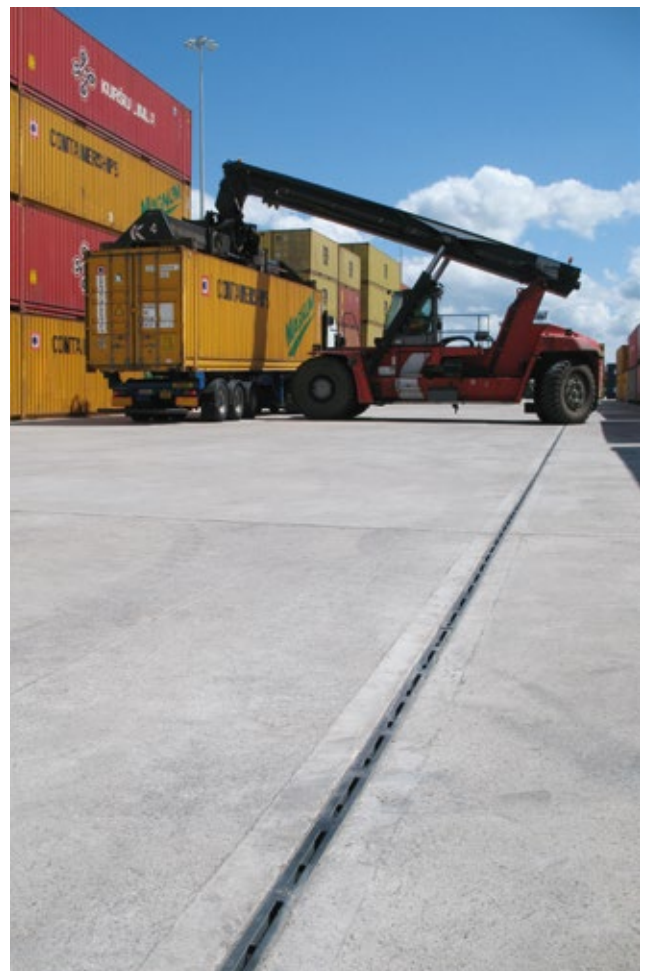
Teesport Container Terminal, UK
