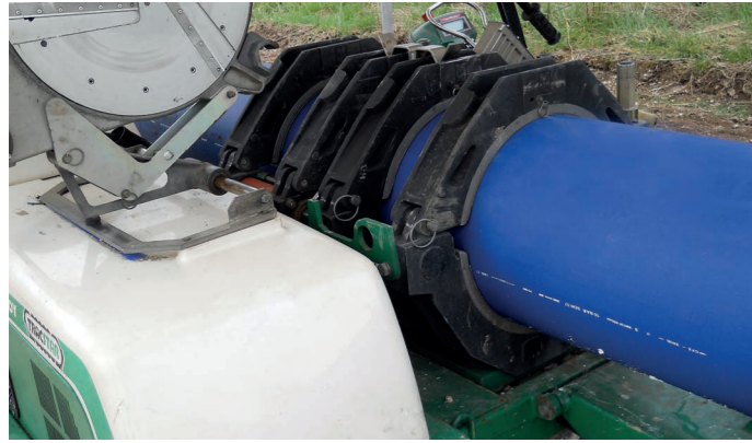
Butt Fusion machine prior to commencement of fusion process
