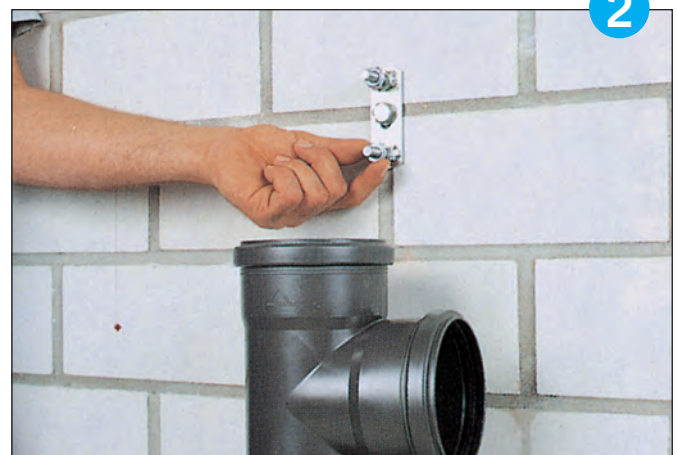
Adjusting the distance from the wall.
