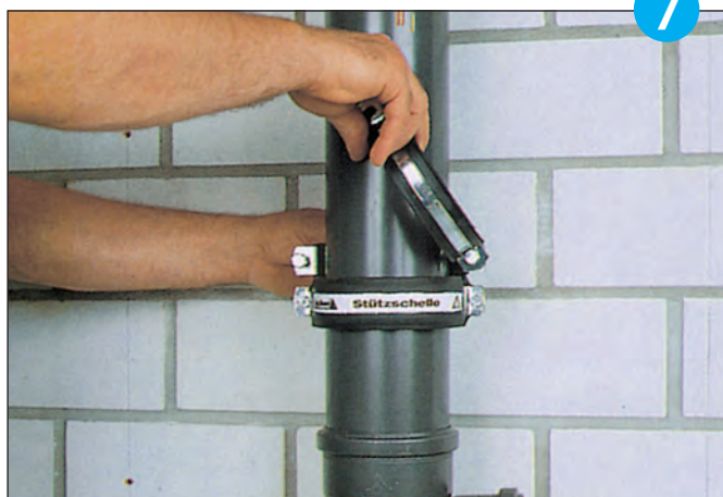
Fix the support ring onto the Friaphon pipe so that it rests on the support clip.
