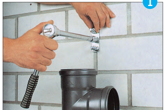
Mark, drill and fit the wall attachment.
