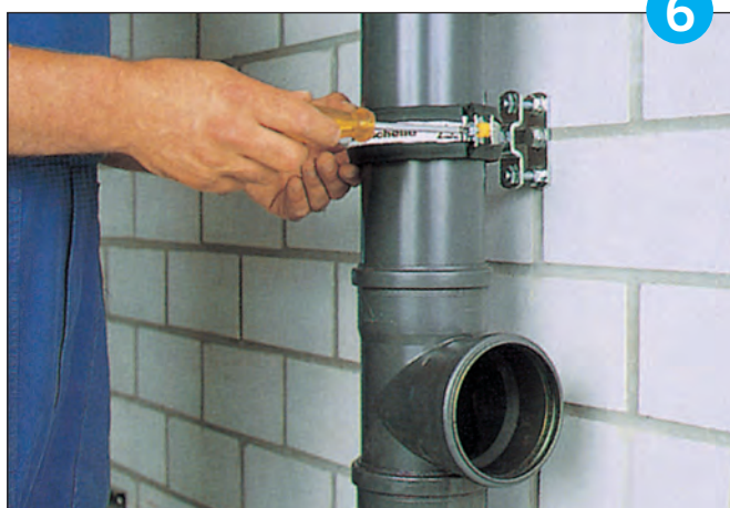
Assemble the support clip and secure the screws on the snap lock. A spacer prevents overtightening.
