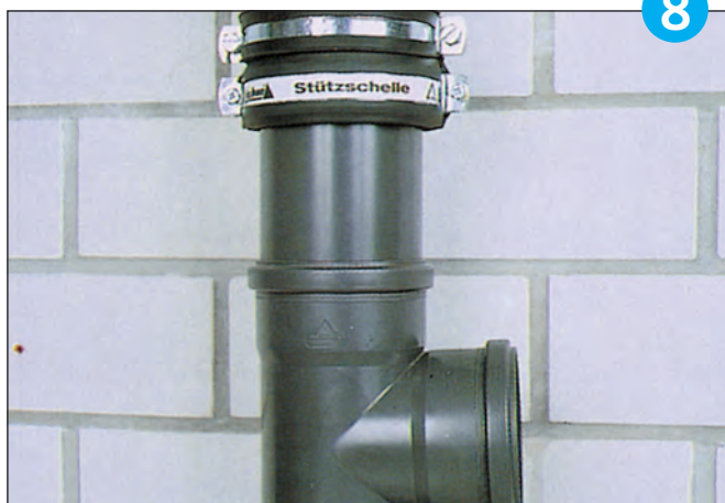
Finished assembly of the complete Friaphon support clip.
