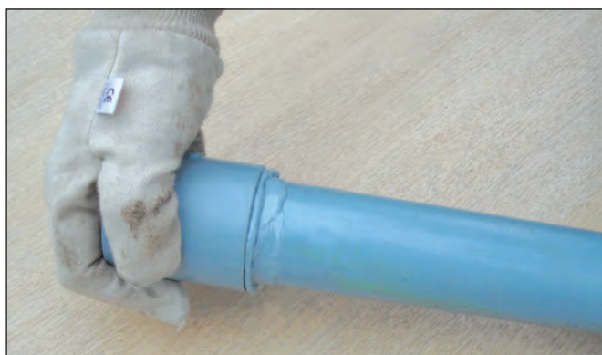
10. Push fitting home and hold for a few seconds.
