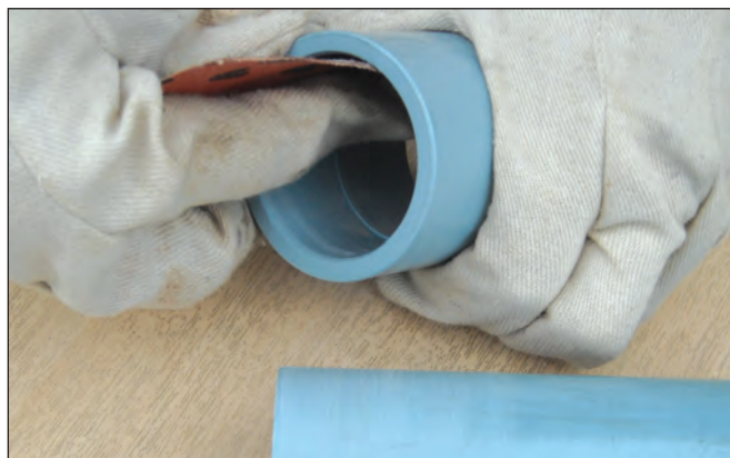
4. Abrade pipe and fitting.
