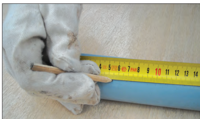
6. Mark on pipe socket depth and a known value.
