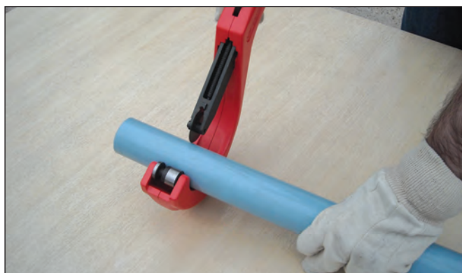
2. Cut pipe to required length.
