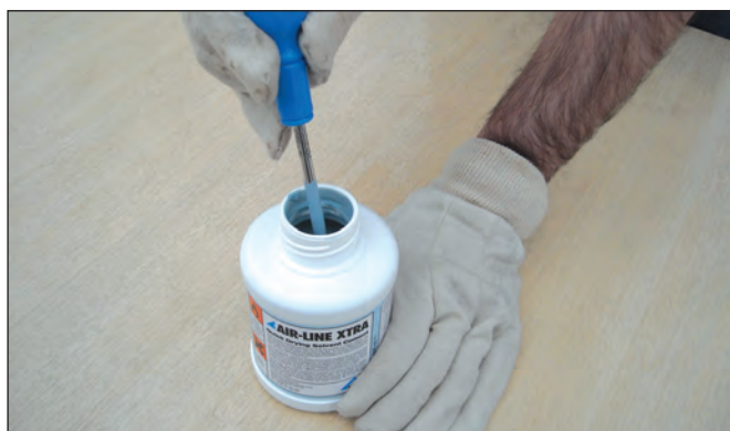
8. Stir solvent cement.
