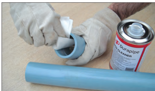
7. Clean pipe and fitting with eco cleaner.
