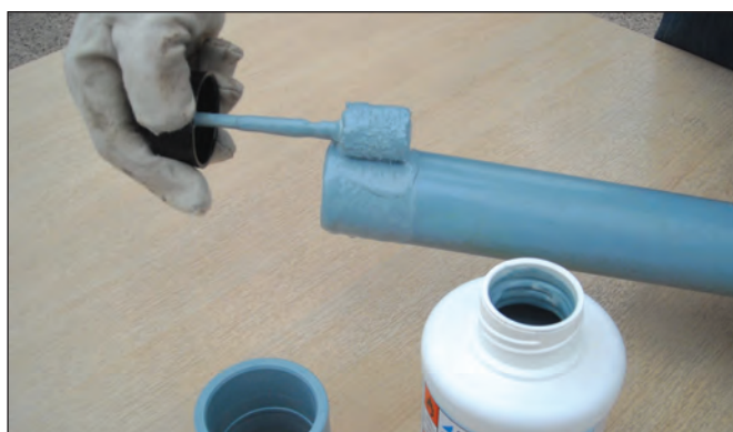
9. Apply cement to pipe and fitting.
