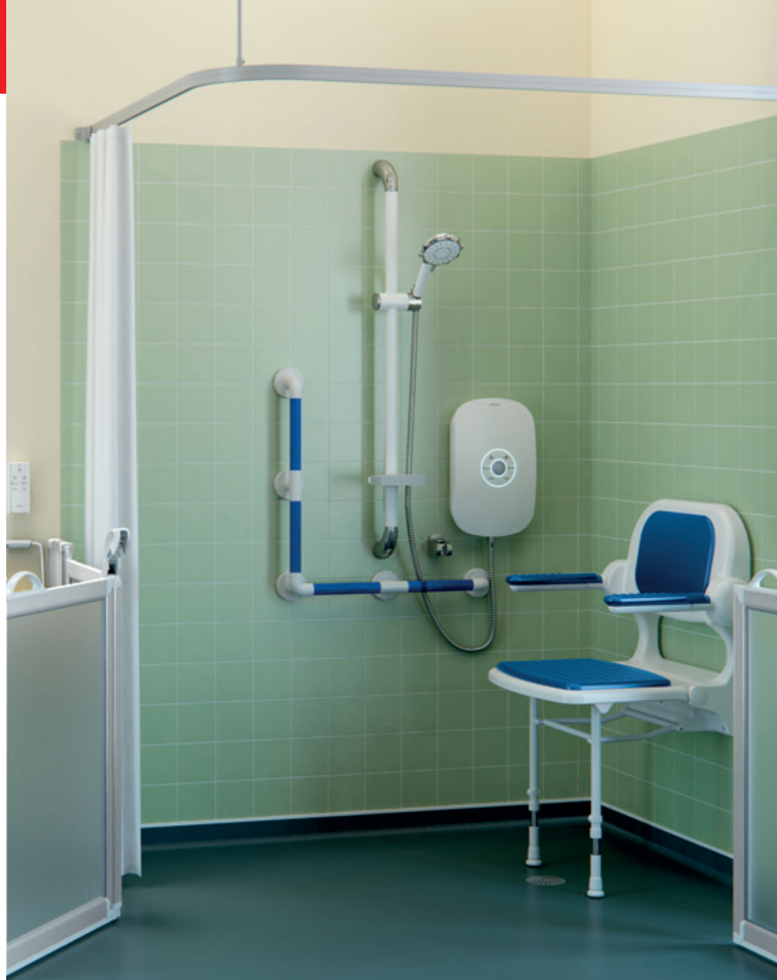
Dementia-friendly bathroom installation by AKW. High contrast blue & white grab rails, shower seat and accessible AKW SmartCare Plus Electric Shower.
