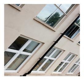
On the first floor of The London Building Centre in Store Street, seven tilt and turn GENEO® windows have been installed to replace 1960s aluminium frames as part of an overall refurbishment programme which is aiming to achieve a BREEAM Excellent rating.
