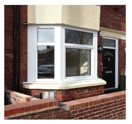
GENEO® windows have been installed throughout a project carried out by Orbit Heart of England Housing Association which aims to maximise the energy efficiency of a traditional 1900s mid terrace house.
