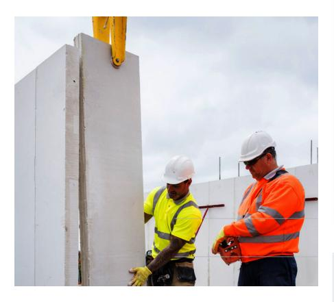
Developed to enhance the key benefits of our thin-joint system; speed and quality of build with reduced waste, H+H UK's Celcon Elements offer all the attributes of aircrete as a building material whilst offering additional value to the project.
