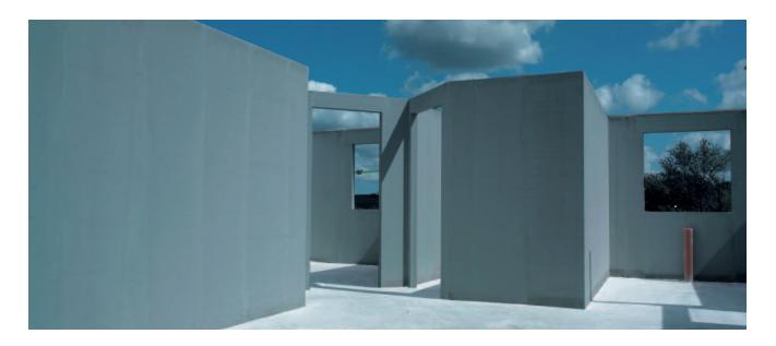
Developed to enhance the key benefits of our thin joint system; speed and quality of build with reduced waste, H+H UK's Vertical Elements (100) offer all the attributes of aircrete as a building material whilst offering additional value to the project.
