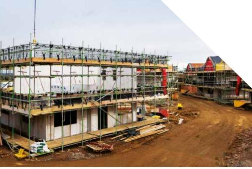
Celcon Elements are manufactured to the design storey height of the house with a width of 600mm and a thickness of 100mm. Elements are craned into place onto a bed of mortar on standard foundations. Vertical joints are filled with H+H element mortar – a fast-setting and very strong thin-layer mortar developed especially for use with the Elements and which forms a 2mm airtight joint.
