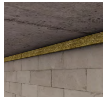
Figure 1 Linear Firestop 2A
