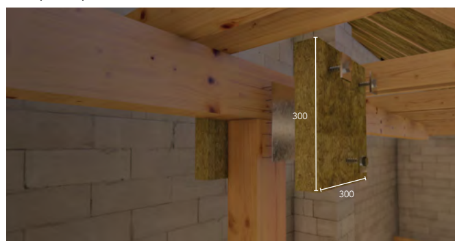
Figure 9 Nail plate protection
