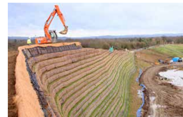
ParaGrid® wrapped-face noise bund at Gatwick Airport
