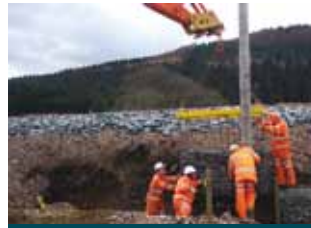
Dalguise, Perthshire, Installation of Prefilled Gabions
