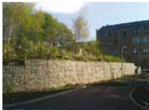
Glencloy Road, Glasgow, Gabion Cladding
