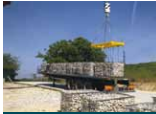
DIRFT, Daventry, Loading of Prefilled Gabions
