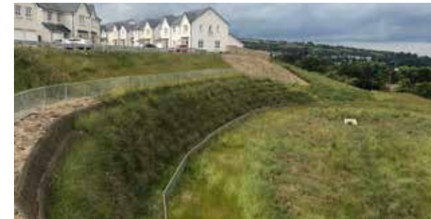
Mineral Terramesh® under construction
