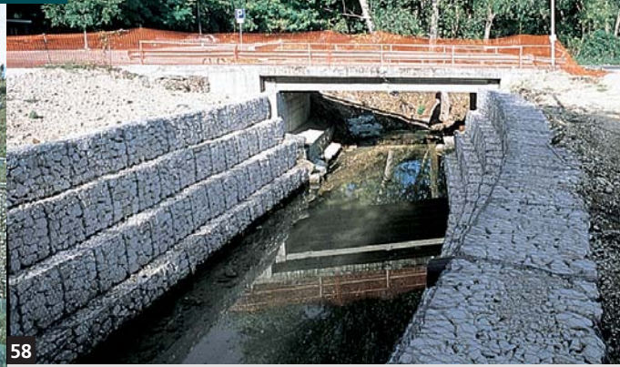
58. Hydraulic protection with Terramesh® S and gabions, Vella river, Sulmona (AQ)-Italy.
