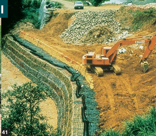
40-41. Slope stabilization with geogrids, Tapei-Taiwan.
