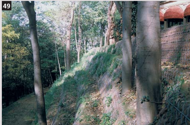
49. Green Terramesh® retaining structure, Bologna-Italy.
