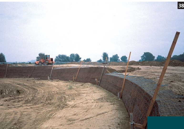
38-39. Green Terramesh® retaining wall, Civitanova Marche (MC)-Italy.
