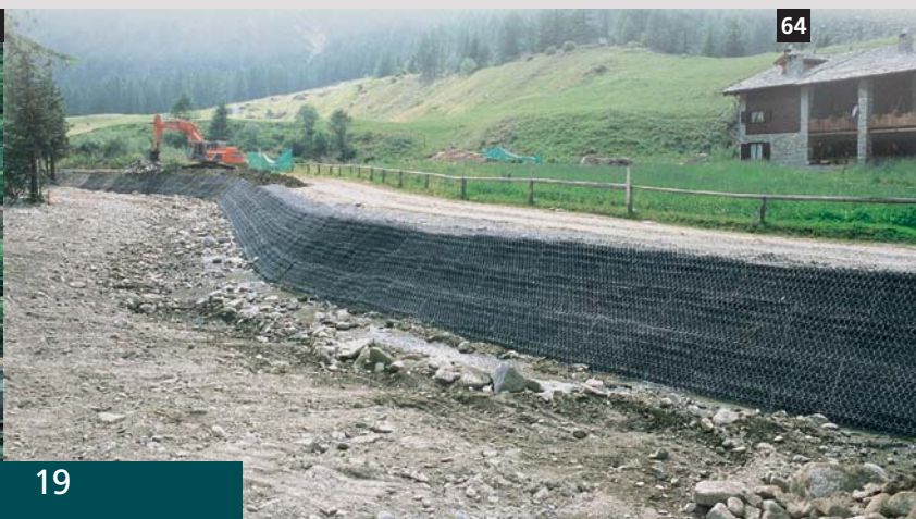
64. River bank protection with Green Terramesh® Water, Cogne (AO)-Italy.
