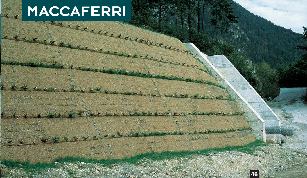
45-46. Retaining wall and hydraulic works with Green Terramesh® Water, Ugovizza (UD)-Italy.
