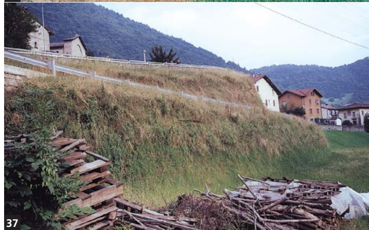
35-36-37. Road restructuring using Green Terramesh®, Valle d'Ogna (BG)-Italy.
