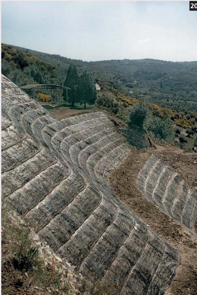
20-21. Slope stabilization in geogrids, Passignano (PG)-Italy.
