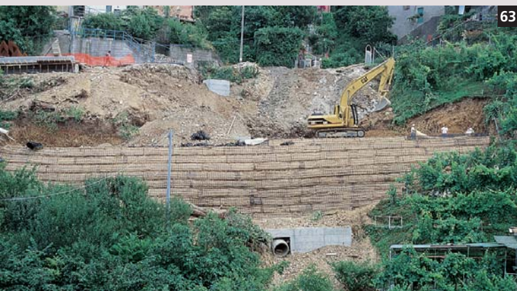
63. Geogrids retaining structure for enlargement of a road, Arcola (SP)-Italy.
