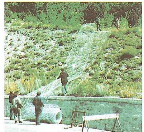
■ ITALY - Valle D'Aosta Erection of netting carried out manually.
