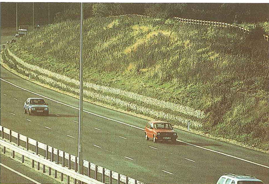
■ ENGLAND - Buckinghamshire M40 motorway widening between junctions 4 and 5. Approximately 5.5km of gabion walling.
