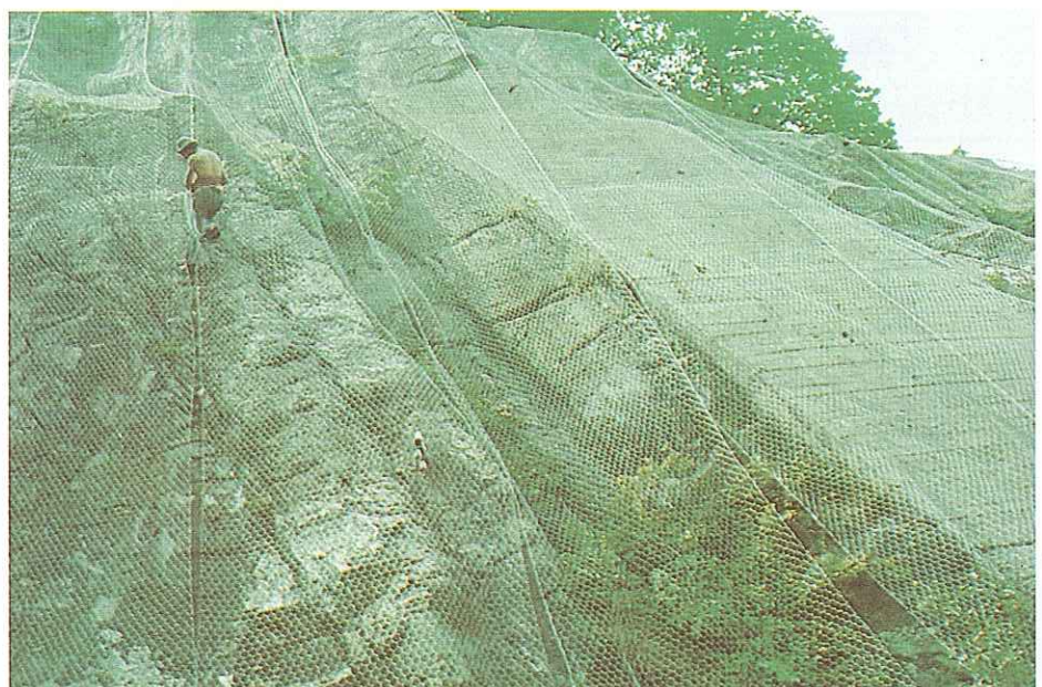
■ ITALY Lacing the netting.
