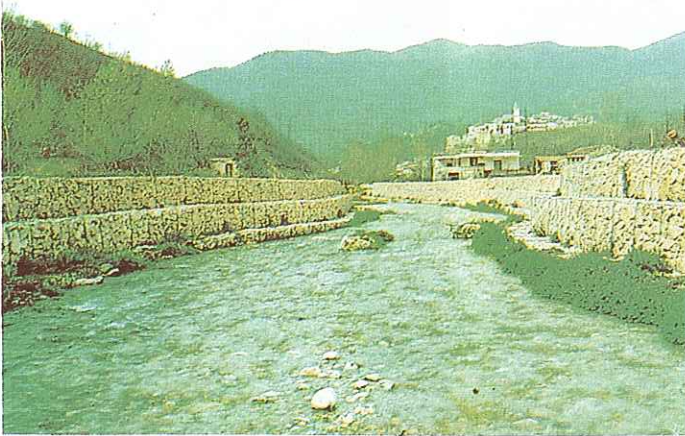
■ ITALY - Campania Longitudinal walls on River Lete.
