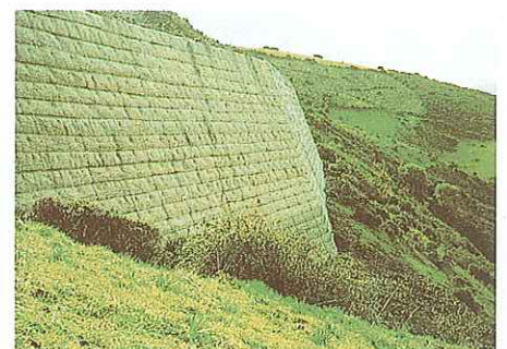
■ ITALY - Sardegna Retaining works carried out with Green Terramesh® units along the road Bitti-Lula which connects the SS131 to the SS389.
