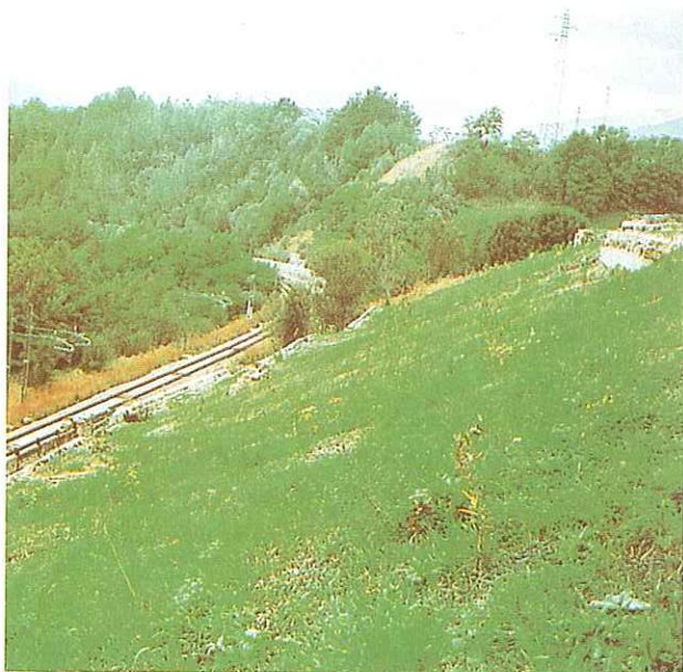
■ Italy - Trentino-Alto Adige Protection with MacMat-R® of slope overlooking a railway in Brunico-Bolzano, near Perca (BZ).
