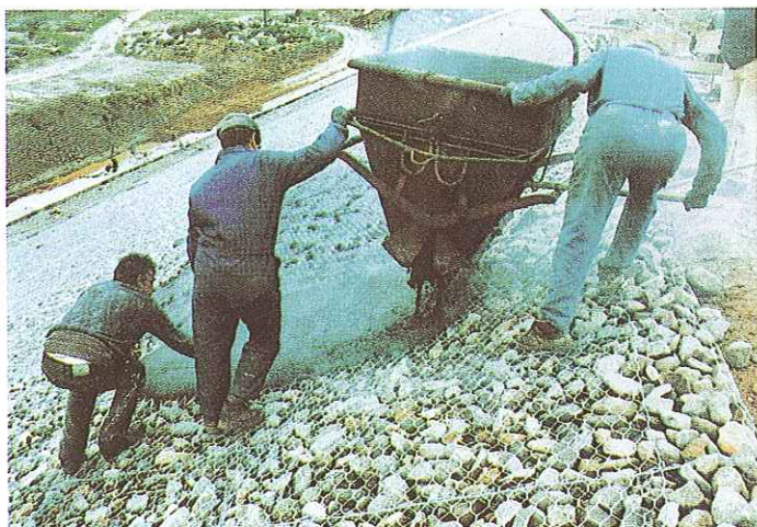
■ ITALY - Sardegna Lochele dam (Nuoro) Reno® mattresses can be sealed by hot poured sand asphalt mastic, in order to provide an impermeable revetment.
