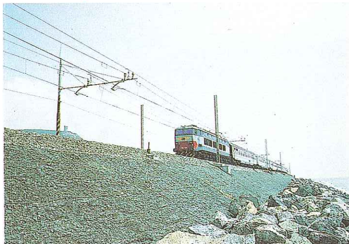
■ ITALY - Calabria Reno® mattress lining carried out along the railway line Salerno-Reggio Calabria near Amantea (CS).
