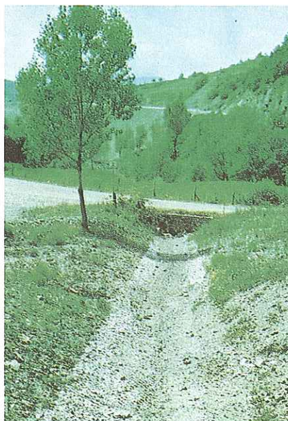
■ ITALY - Tuscany Drainage channel to stabilise a slope near Florence.
