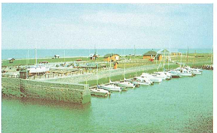
■ CANADA - Quebec Marina walls at Matane; the work was carried out using PVC coated gabions.
