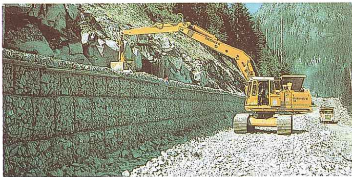
■ Gabion filling operation.
