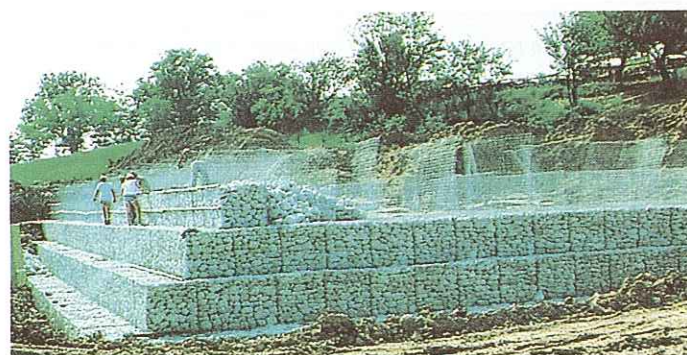
■ Reno® mattresses filling and closing operation.
