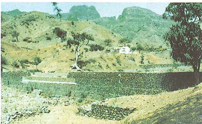
■ REPUBLIC OF CAPE VERDE Series of structures for soil conservation on Santiago Island.
